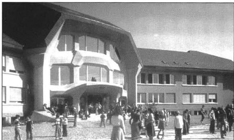
Figure 39. Front Facade, Rudolf Steiner School, Ittigen.
